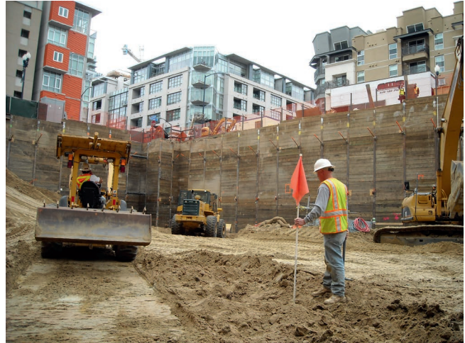
Figure 4. Pat Sena monitoring excavations into Middle Pleistocene deposits of the Bay Point Formation at the Thomas Jefferson School of Law project site, downtown San Diego, California.
