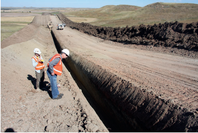
Figure 5. Georgia Knauss operates a Trimble GPS receiver while Dale Hanson examines rocks of the Sentinel Butte Formation (Fort Union Group) exposed in a natural gas pipeline trench in North Dakota.
